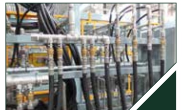
Hidrolik Tesisatlama Hydraulic Installation
